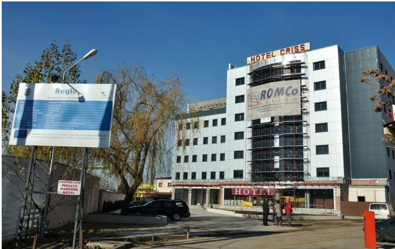
Extindere Hotel Criss-Bucuresti
